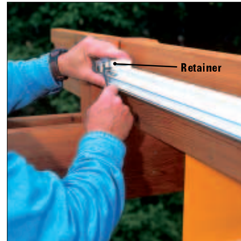
5 Install the retainers on the track at the saddle beam.
