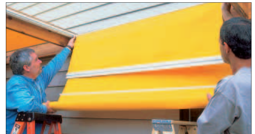
6 Feed the canopy rollers into the tracks at the ledger, starting with the outermost cross member's handle end.
