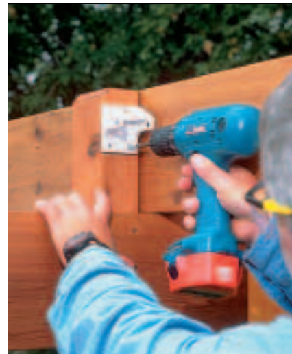
2 Mount the corresponding track brackets to the vertical braces above the saddle beam.
