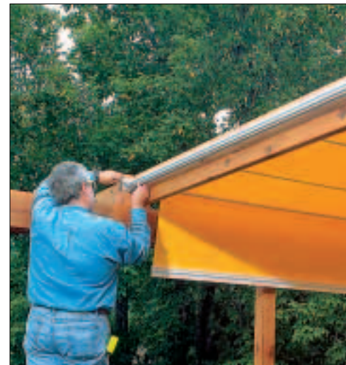
3 Slip the track over the extender and secure the outer end to the brackets (as shown).
