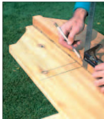
**3** After laying out the positions of the joists on the ledger, transfer the marks to the tops of the beams using a combination square.
