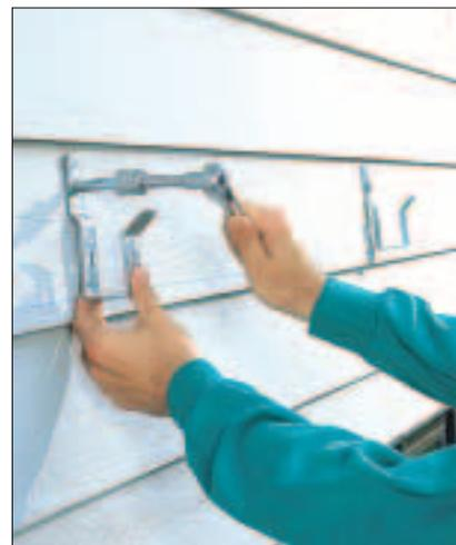
**5** Predrill and bolt the Stratton brackets to the house to support the ledger board. Position the brackets so you drill into solid house framing.
