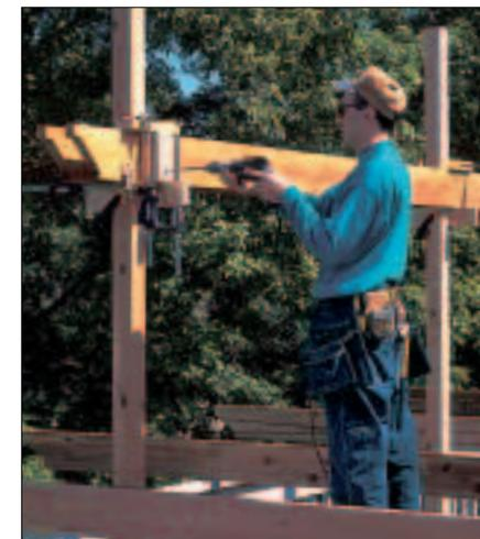
**7** Temporarily clamp the pergola's saddle beam to the post and predrill for bolts. A simple wooden alignment jig ensures uniform and straight holes.
