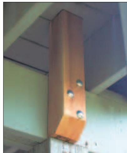
**6** Secure each post to the deck's main support beam with three 1/2 x 12-in. carriage bolts; or strap and toenail the posts to the top of the beam.
