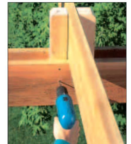
**10** After checking the joist assembly for square, secure the free ends by mounting pairs of vertical blocks with deck screws between the beams.
