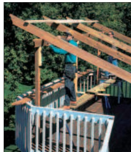
**8** Lift the beam and the free ends of the joists simultaneously and rest the beam on support blocks for bolting. Note the temporary bracing.
