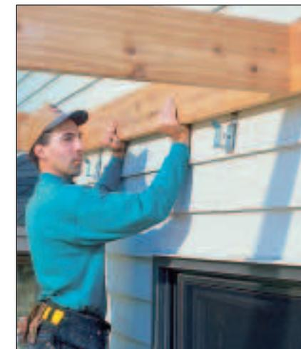
**9** Mark the Stratton bracket positions on the ledger to ease alignment, raise the joist assembly and slip the ledger into the brackets for bolting.
