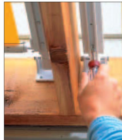
**4** Fasten the tracks to the extenders at the ledger end.
